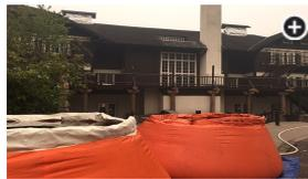
Structural protection specialist Kevin Smith tells us one way of prevention is using structural wraps. The wrap comes with an aluminum side and a cloth side. The shiny aluminum is there to reflect heat from potential nearby flames away from the building. The other thing wrapping does is prevent embers from jumping into the vents.
